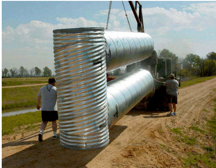
Figure 6. U-tube prior to installation. The tube was 35" I.D. x 20' tall and was made with 14 gauge galvanized steel.
