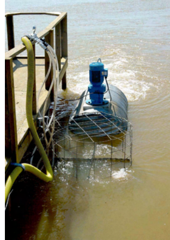
Figure 8. As the water level dropped below the top of the culvert (as shown in this photograph) flow decreased; if water level rose above the top of the culvert the motor could be damaged.
