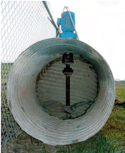
Figure 7. View into the discharge end of the tube, showing the impeller, shaft, and motor (mounted on top).
